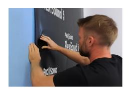
**8.** Install FlexiSound. FlexiSound is self-adhesive and requires no fixings or secondary adhesive. Stick the FlexiSound to the plasterboard covering the entire wall leaving no gaps. The FlexiSound can touch the walls and ceiling, as it is a soft material and won't aid in the transfer of sound energy. It also helps to seal the first layer of plasterboard.
