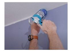
**10.** Finally, remove the shims and fill the gaps around the perimeter with Acoustic Sealant.
