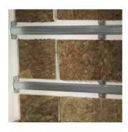
**4.** Install 25mm Acoustic Mineral Wool between bars and affix using Contact Spray Adhesive. No need to cover the whole wall, there can be gaps (as per the image opposite). Ensure the acoustic mineral wool doesn't touch the furring bars (it can touch the clips).
