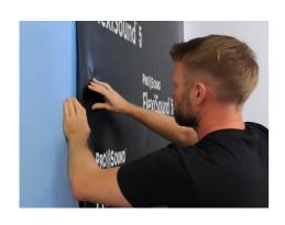
**8.** Install FlexiSound 5. FlexiSound is self-adhesive and requires no fixings or secondary adhesive. Stick the FlexiSound to the plasterboard covering the entire wall leaving no gaps. The FlexiSound can touch the walls and ceiling, as it is a soft material and won't aid in the transfer of sound energy. It also helps to seal the first layer of plasterboard.
