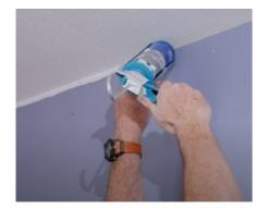
**10.** Finally, remove the shims and fill the gaps around the perimeter with Acoustic Sealant.
